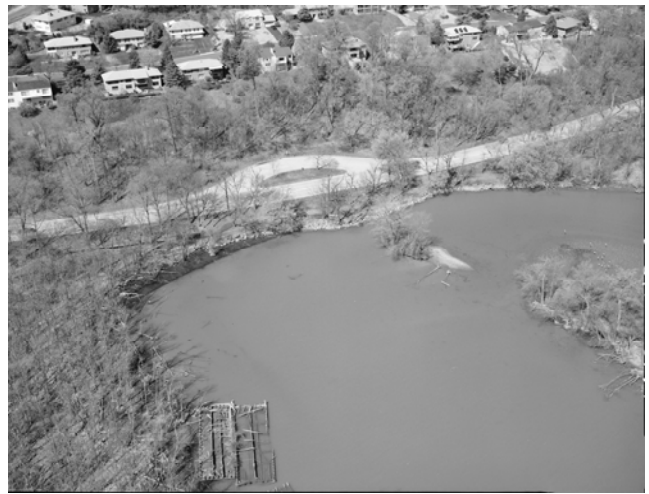
Dyke Marsh Pull-off aka Cigarette Turnaround. The photo is from the National Park Service Historic American Building-Historic American Engineering Record Survey.
